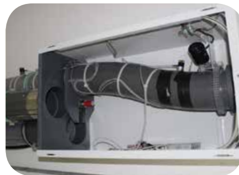
THE 3-WAY DIVERTER TO ENABLE MULTIPLE ITEMS TO BE SENT & RECEIVED VIA P.T.S.
