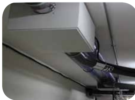
THE 3-WAY DIVERTER TO ENABLE MULTIPLE ITEMS TO BE SENT & RECEIVED VIA P.T.S.
